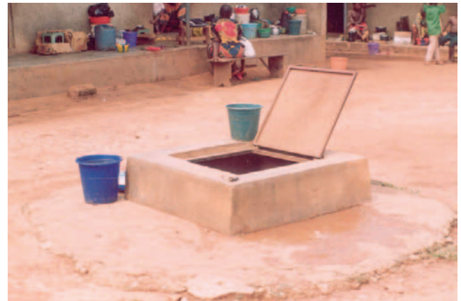
Fig. 2C. A hand-dug well in the courtyard, the main source of water for the centre.
