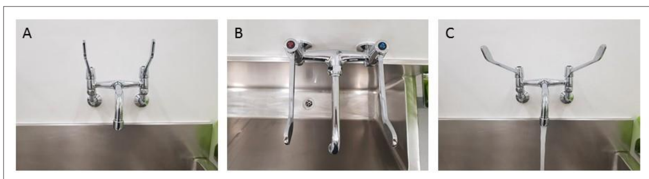
Fig. 1. Adjusted tap levers in the closed position (A and B) and the open position (C).
